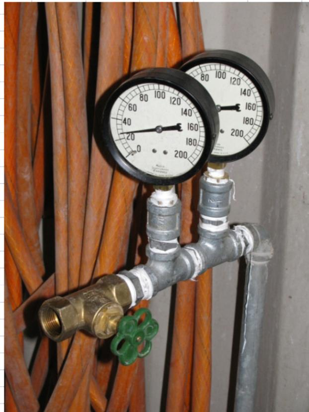
Note: pressure test pump connection shall be made to the inlet tee (run ) using threaded connection from the pump
